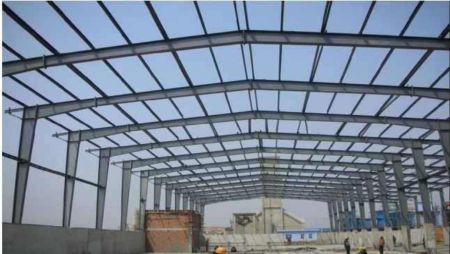
Industrial building under construction
